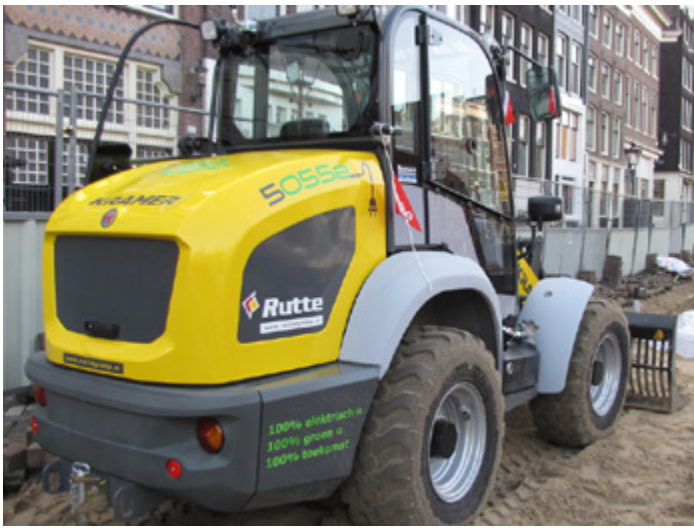
An electric shovel in Amsterdam's city centre (credit: AT5)
