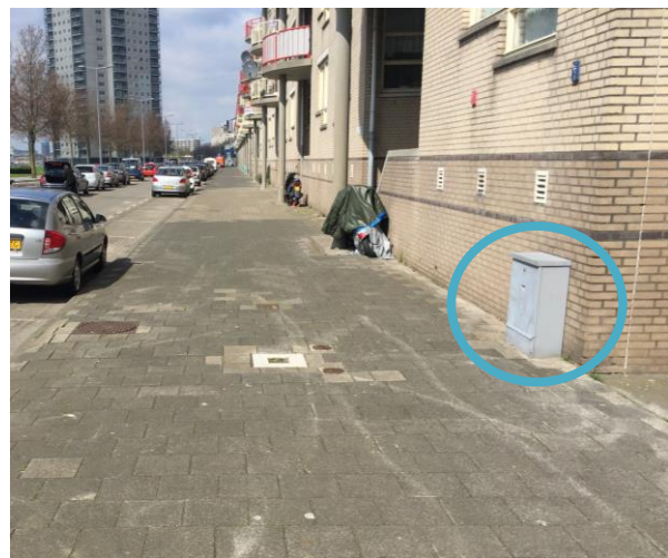
Figure 13: Example of the connection for a pumping station in Rotterdam.
