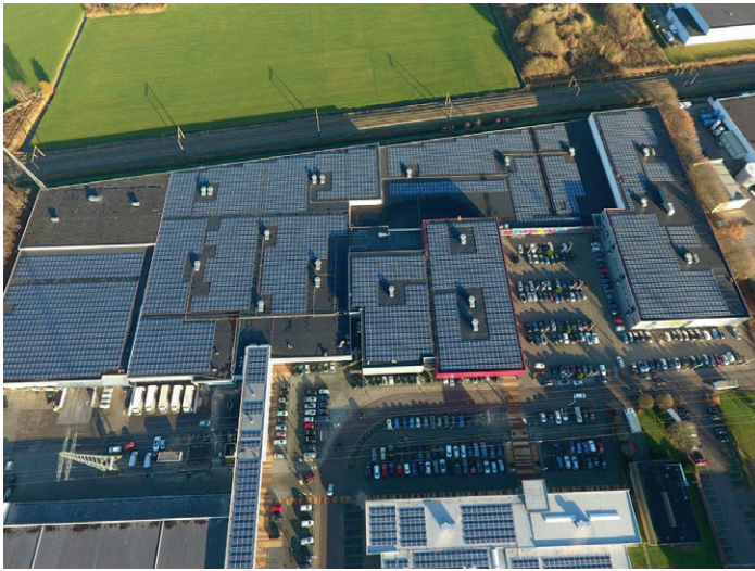
Charging points in the Home Center car park (Photo: GroenLeven)
